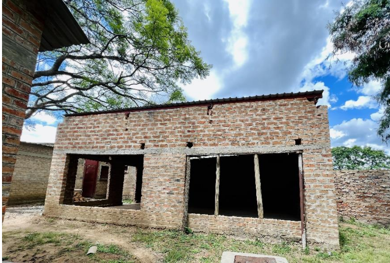
Classroom in progress
